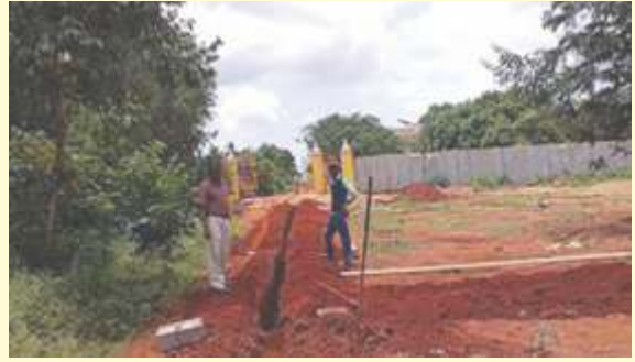
laying of water lines
