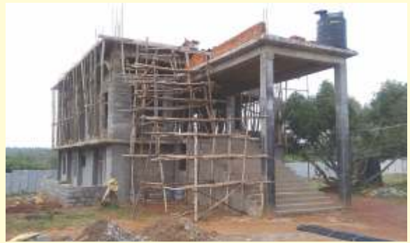
Vihara building under construction
