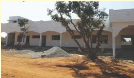
Dining block under construction
