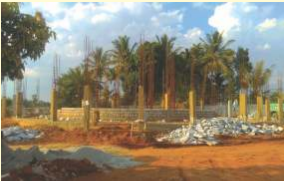
Pagoda under construction April 2015
