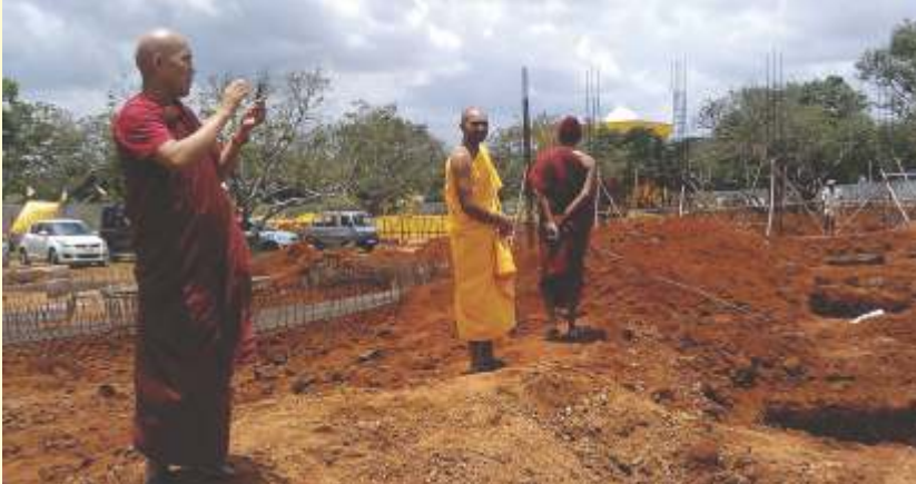
Kassapa bhanteji inspecting the construction
